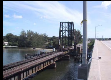
Loxahatchee River FEC RR Bridge
