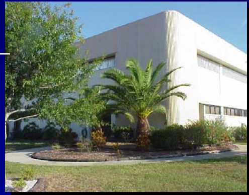
South County WTP (Oslo Road)
