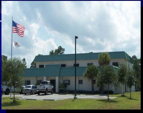
North County WTP (Hobart Park)
