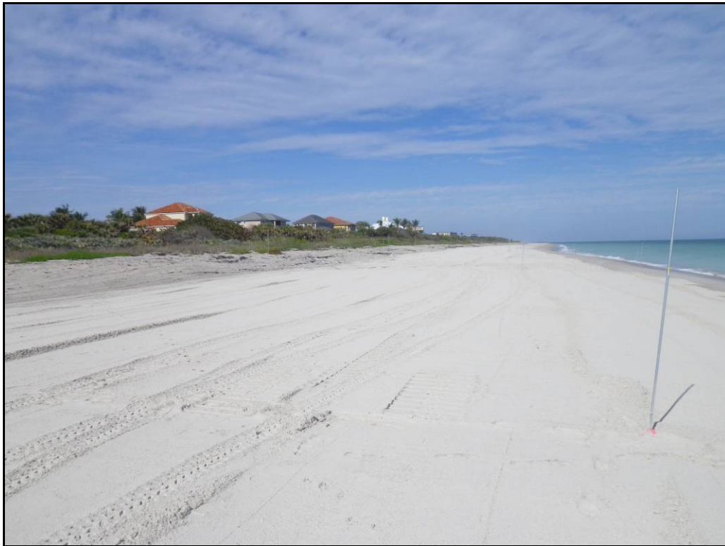
Completed Project Location: Southern Seaview Development - Photo Taken 1-13-12
