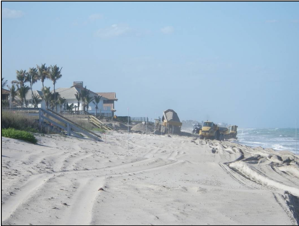
Location – north Windsor area looking north – Photo Taken February 28, 2011
